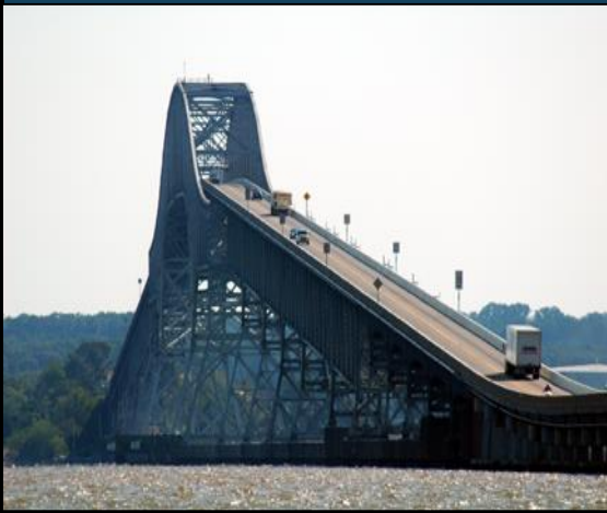
Harry Nice Bridge
